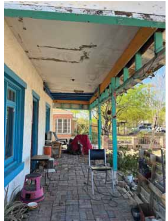
Detail of front porch (view looking south) showing layer of bricks on top of original concrete porch deck. Deficient spliced 2 x 4 porch supports, missing fascia, and damaged porch ceiling are also visible.
