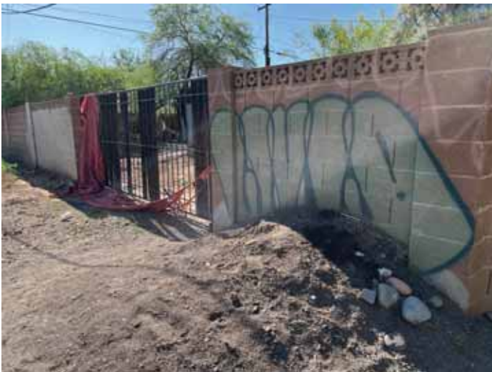
Exterior graffiti and mounding of soil, gravel, and debris to preclude vehicular access to the public alleyway (negatively impact neighboring properties on the north side of the alleyway) and inoperable rolling gate to the rear yard of the property (view looking southeast from the public alleyway).
