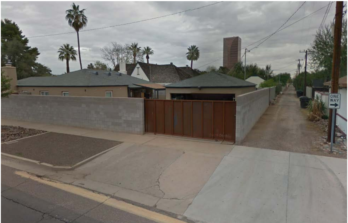
View looking northeast – Google Street View showing 6.8' fence at left (an extra block course and cap), 6.5' gate, and 7.3' alley fence (two extra courses and cap), all unpermitted (February 2017)
