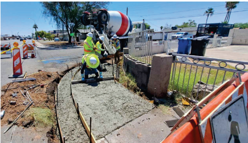
Construction crews are installing hundreds of ADA curb ramps throughout the city, eliminating barriers to mobility for people with disabilities.
