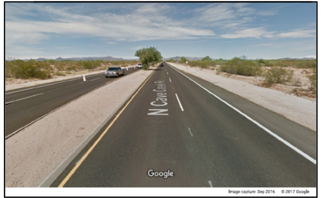
Cave Creek Rd North of Jomax Road Facing North
