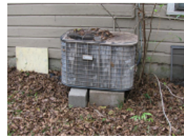
HVAC: The building has broken, detaching, and/or rusted out heating and cooling units, including the evaporate.
