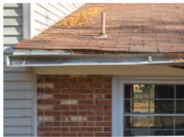
Gutters/Drains: The gables or roof gutters or drains are broken, cracked, or deteriorated in some way.
