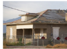
Roof Shingles: The buildings roof shingles are deteriorated. Missing, lifting, curled, cracked, buckled or spotted roof shingles constitute deterioration.
