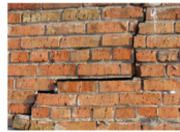
Brickwork: The structural brickwork is eroded, cracked, or missing altogether.
