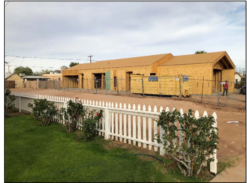
Photo 2. View of subject property, looking northwest from adjacent property.
