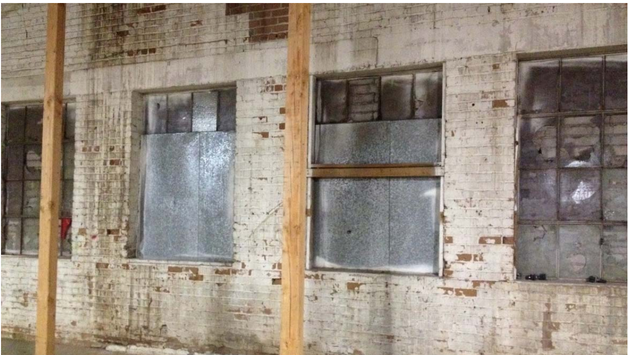
Photo 4. Infilled windows from interior, prior to rehabilitation (2016).
