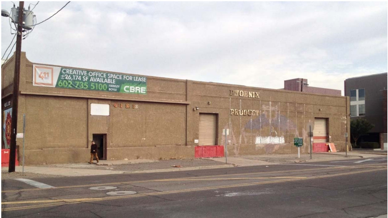
Photo 1. View of west façade of 411 South 1 st Street depicting infilled windows and stucco sheathing, prior to rehabilitation, facing southeast (2016).
