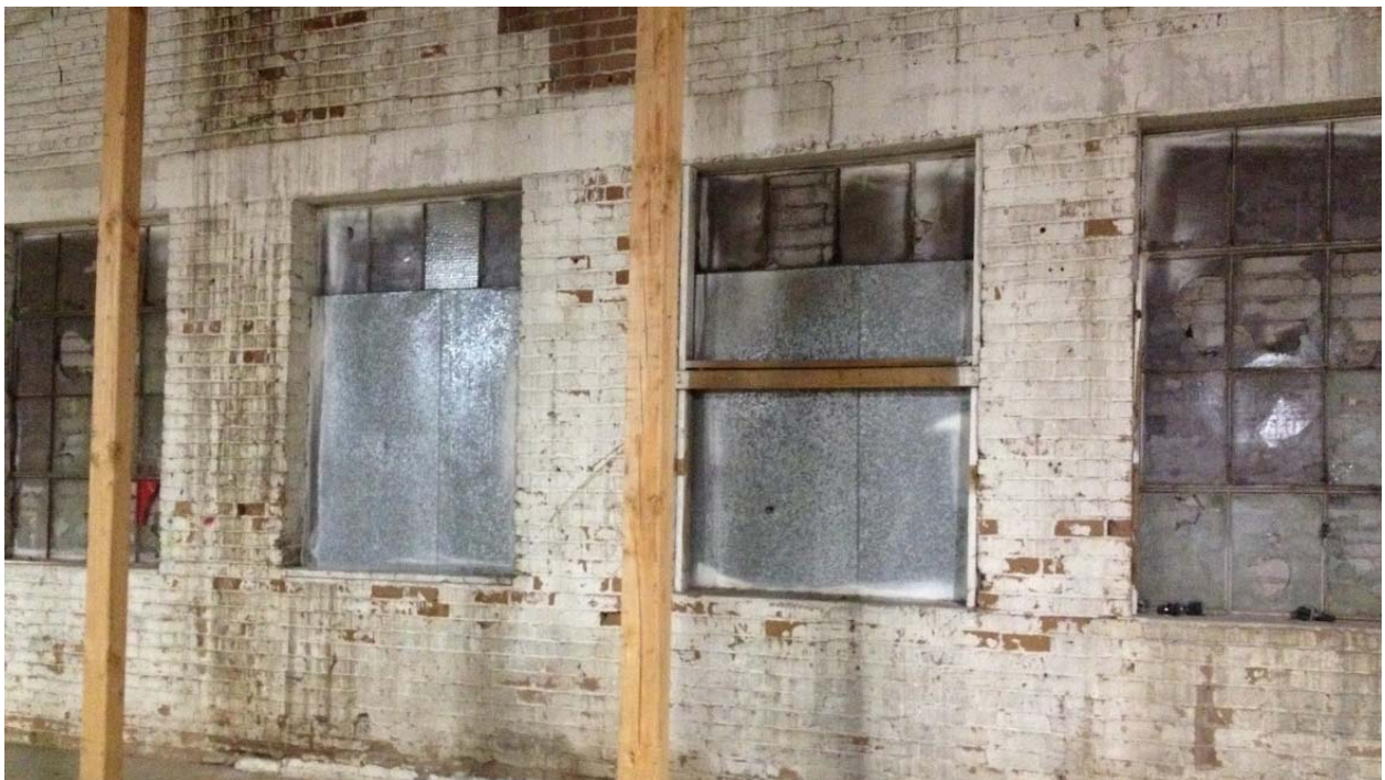
Photo 4. Infilled windows from interior, prior to rehabilitation (2016).
