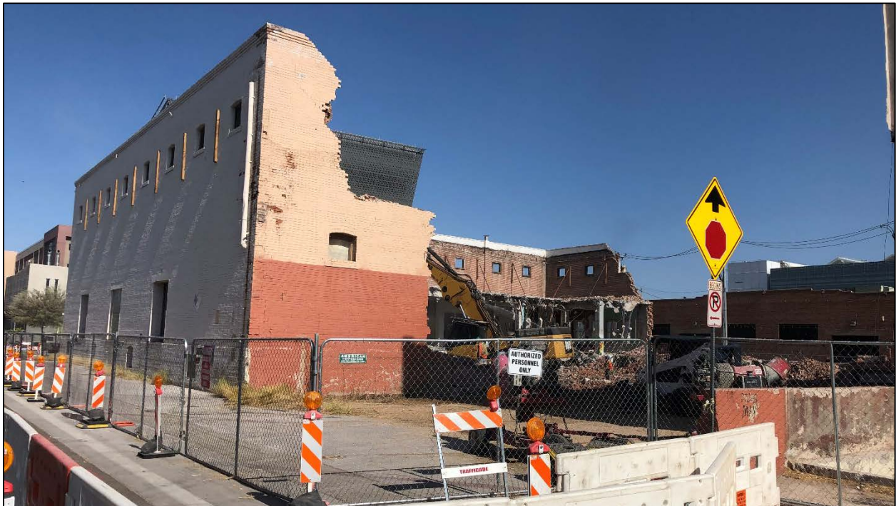
Photo 4. View of demolition in progress, looking northwest from Jackson Street, July 2020.
