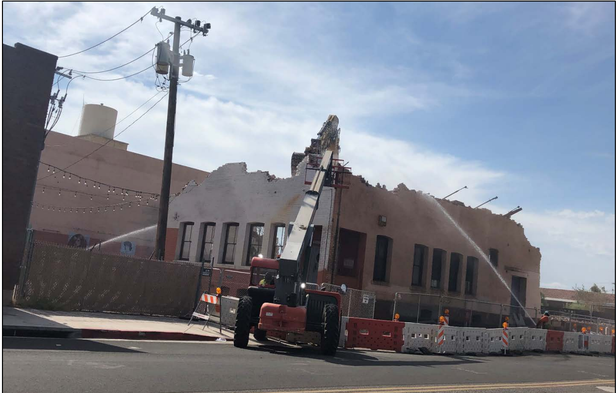
Photo 3. View of demolition in progress, looking southeast from 5 th Avenue, July 2020.
