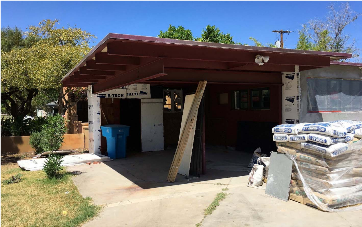
View looking northwest – subject property showing stucco in process over wood siding
