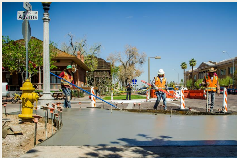
Curb Ramp Under Construction
