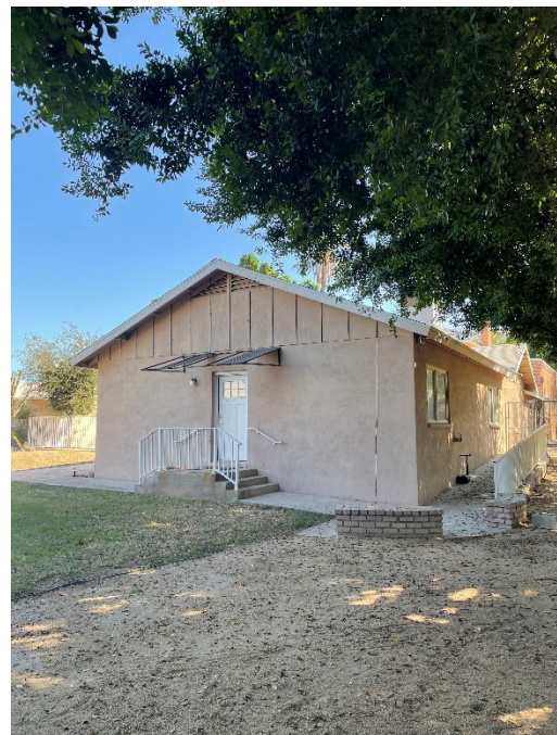
Rear (west) façade of main house, view northeast.
