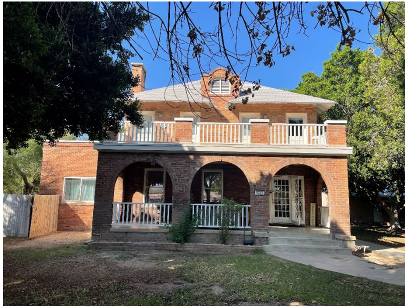
Front (east) façade of main house, view west.
