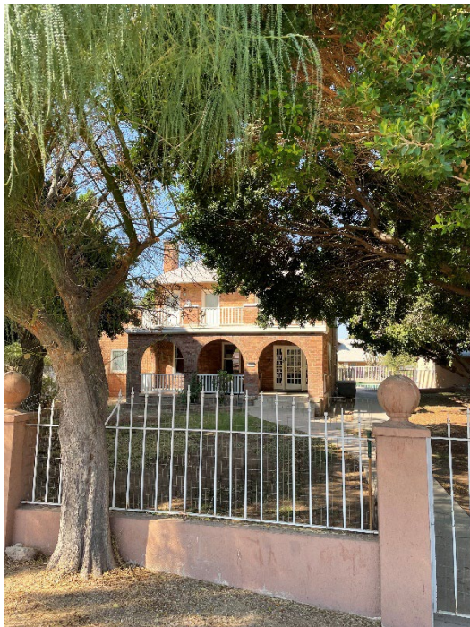
8252 S. 15th Ave. from sidewalk, view west.
