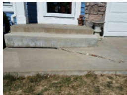
House Walkway: The walkway to the front entry of the building is cracked or missing pavement or pavers.
