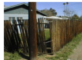
Fence: A part of the fence (alley, front, back, or side) is broken, bent, or has peeling paint.
