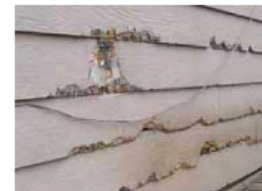
Siding: The siding is missing, bent, or detached.
