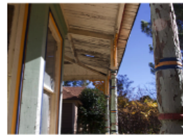
Paint: The paint is peeling or faded, or generally deteriorated.
