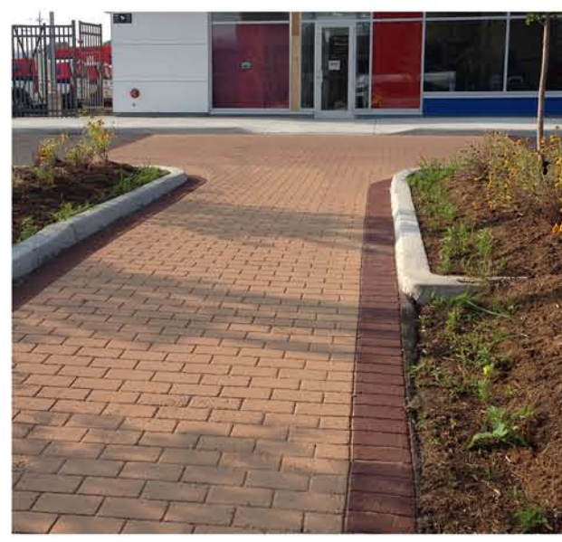
PAVERS AT PEDESTRIAN WALKWAYS
