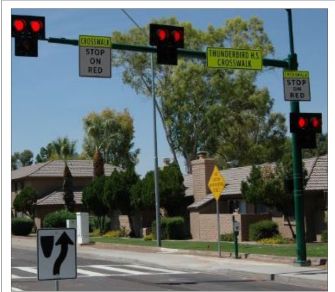
On June 25, 2020, Phoenix's 66th HAWK pedestrian crossing signal was activated at 18th Street and Roosevelt Street. HAWKs make streets safer for people who walk, bike and drive by providing clear alerts when people intend to cross the road.
