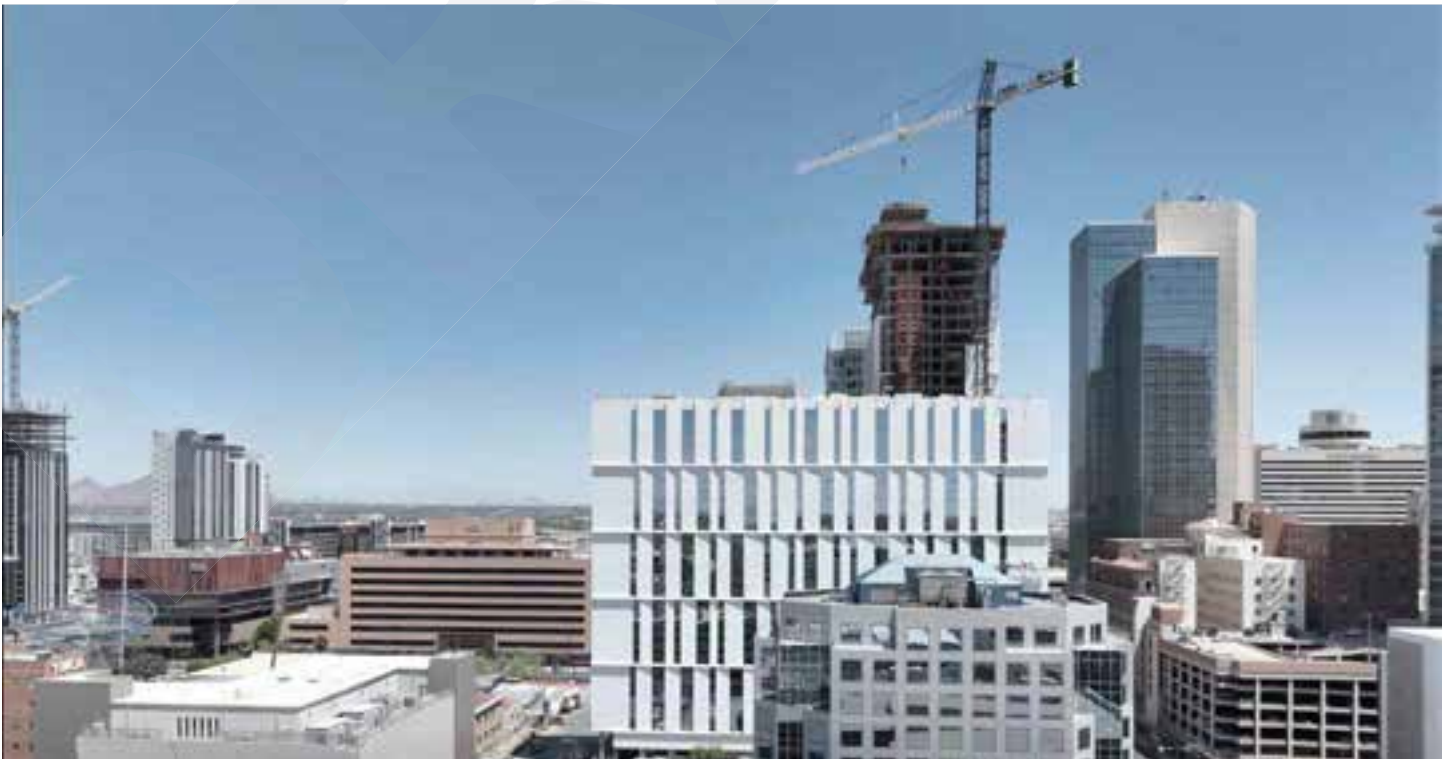
Construction of Downtown Mixed-Use Development - Central Station / Credit: Nick Ryan
