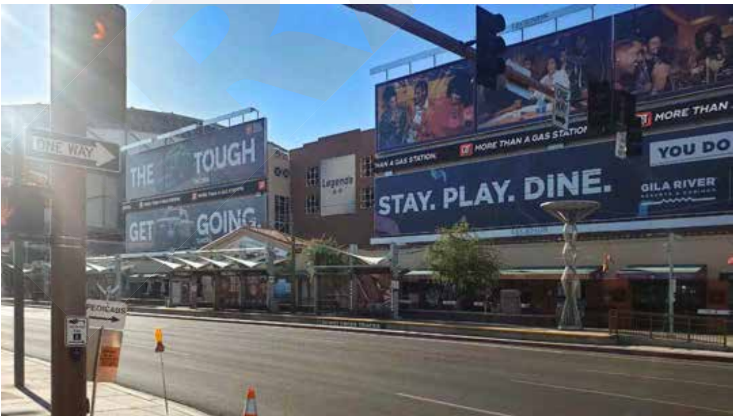
Signage for Billboard Advertisements - Jefferson Street Garage / Credit: Nick Ryan
