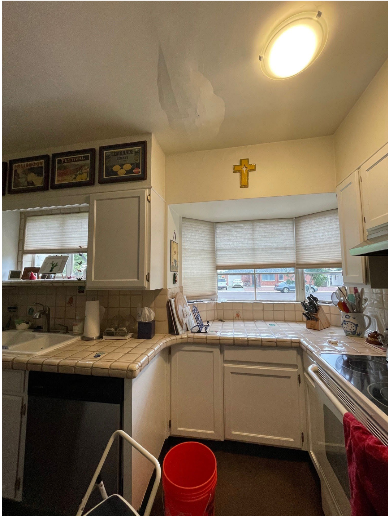
Photo 2. 302 E. Pasadena Ave., interior view. Note evidence of leak in ceiling.
