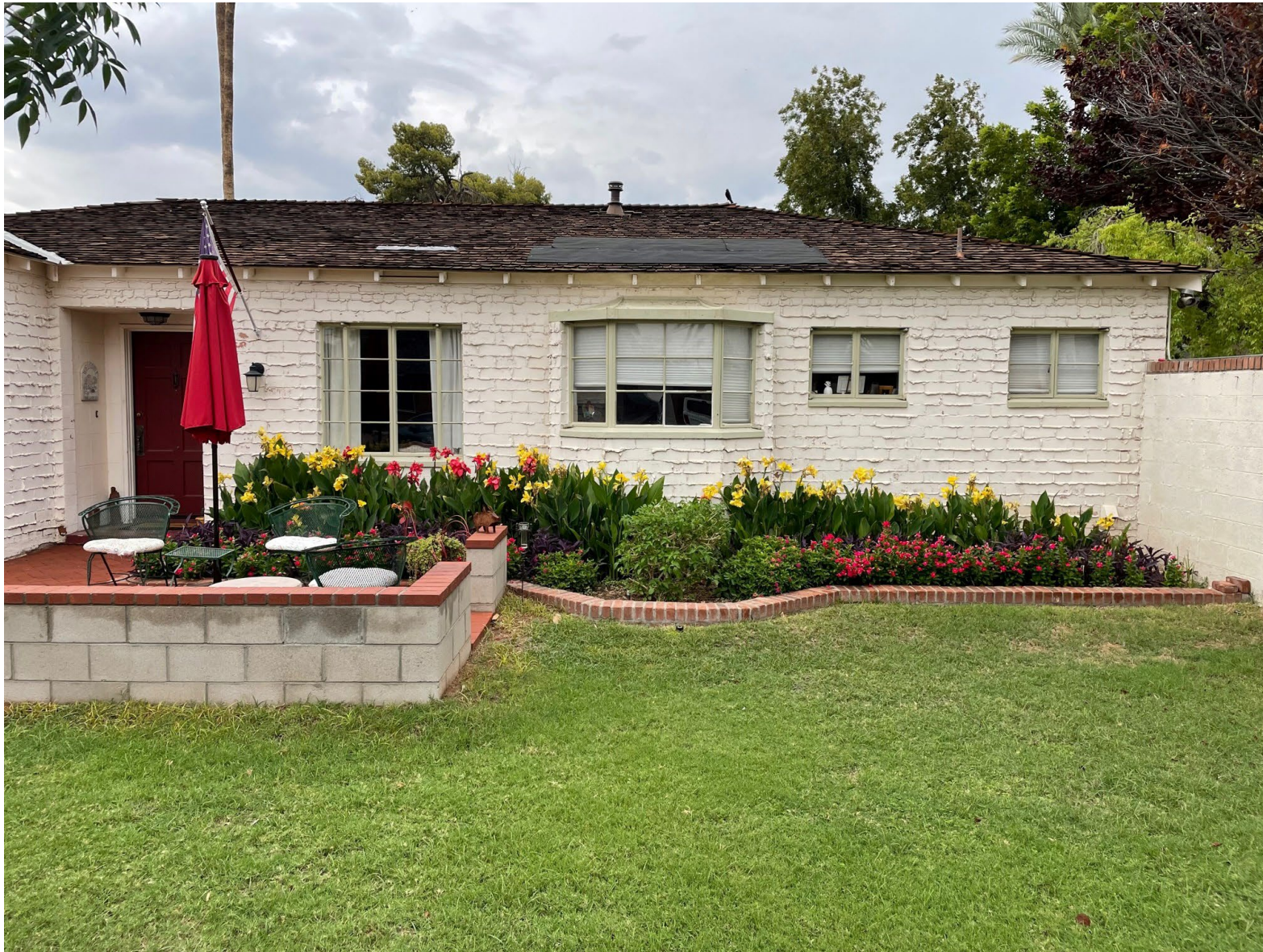
Photo 1. 302 E. Pasadena Ave., front view. Note patch over shingles to address roof leak.
