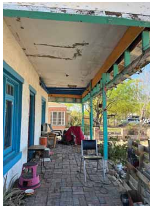
Detail of front porch (view looking south) showing layer of bricks on top of original concrete porch deck. Deficient spliced 2 x 4 porch supports, missing fascia, and damaged porch ceiling are also visible.
