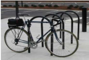
Inverted-U bicycle rack, where both ends of the "U" reach the ground.
