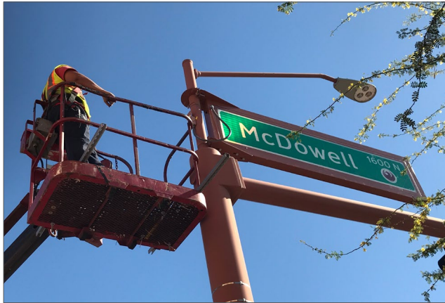
A maintenance crew member works above McDowell Road. As part of technology improvements, signal poles at 440 major intersections were repainted to protect and lengthen the lifespan of the technology housed inside.
