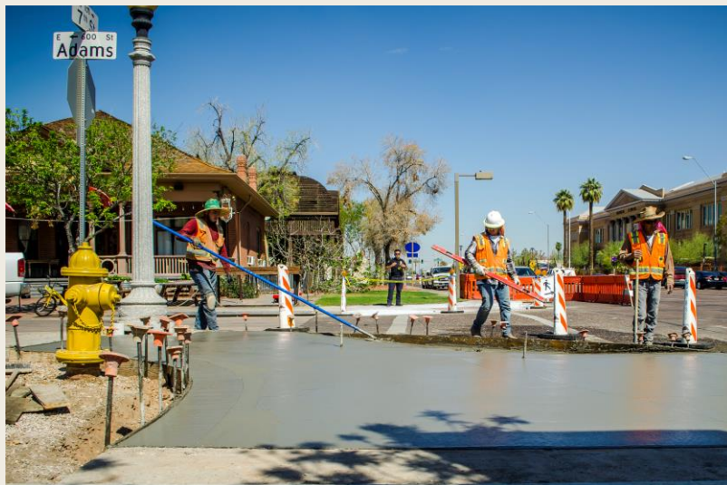
Curb Ramp Under Construction
